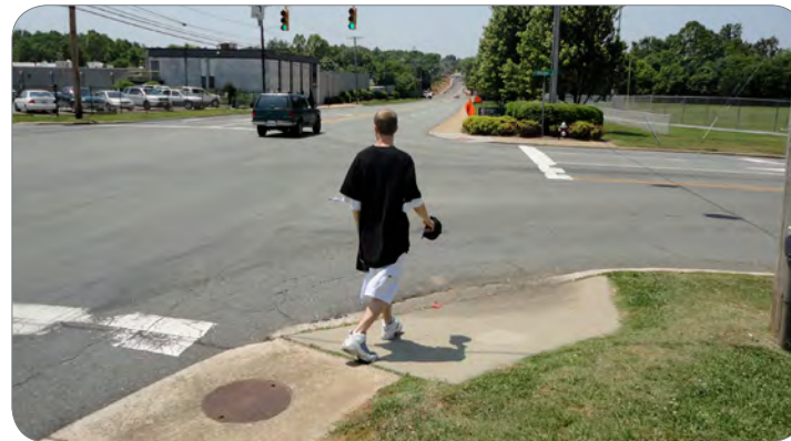
▲ Pedestrian crossing a roadway with poor curb ramps, no marked crosswalk, and no pedestrian signalization in Burlington, NC.
