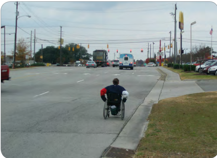
▲ Pedestrian forced to use roadway where sidewalk gap exists in Jacksonville, NC.
